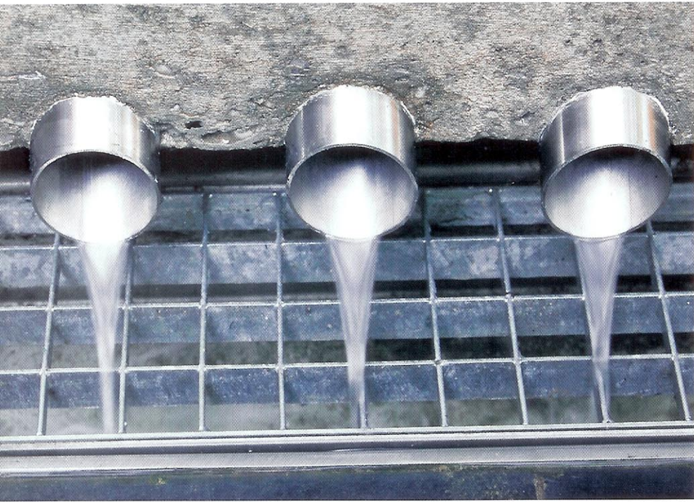
ABOVE: WATER IS PUMPED THROUGH STAINLESS STEEL PIPES TO CREATE A CONTINUOUS FLOW ALONG THE CONCRETE BENCH; THE PURPOSE-MADE GALVANISED STEEL GRILLE PARTIALLY CONCEALS THE WATER AS IT TRAVELS BACK TO BE RECIRCULATED.
